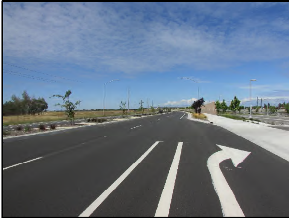
View of subject property looking westerly from near middle of corridor
